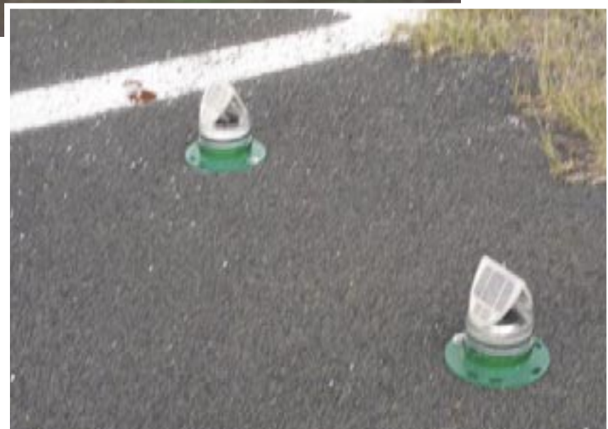
Solar powered emergency airfield lights, RFDS Charleville Base, QLD Australia
