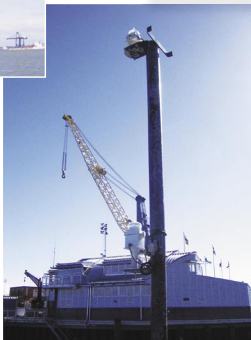
SL10 Dual Pier Lights, Harwich Harbour, United Kingdom
